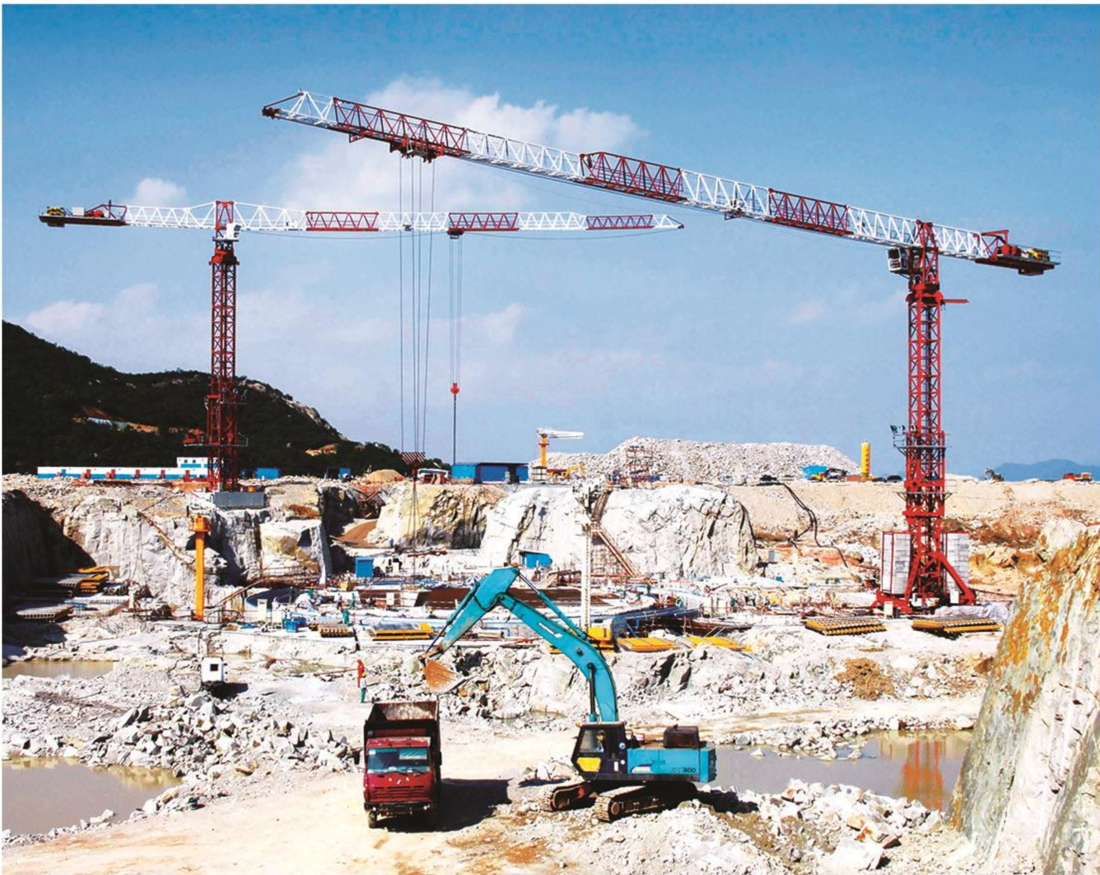
核岛负挖施工 Nuclear island negative excavation construction
