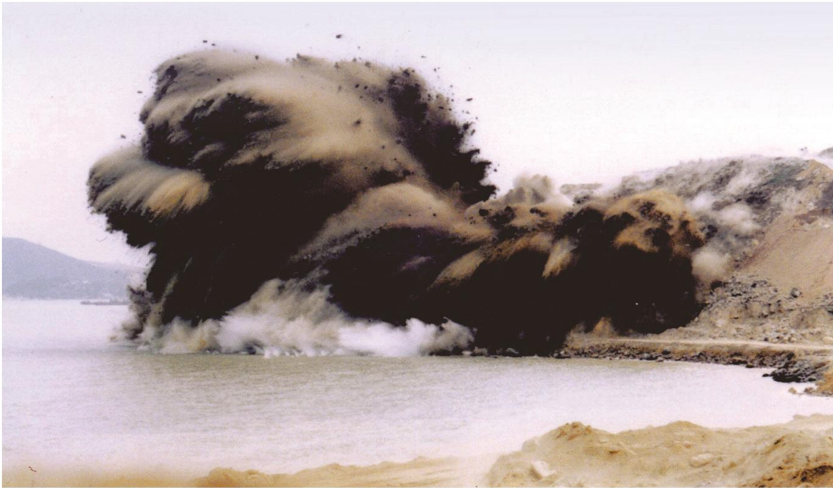
大型土石方爆破预控技术 Large-scale earth and stone blasting pre-control technology
