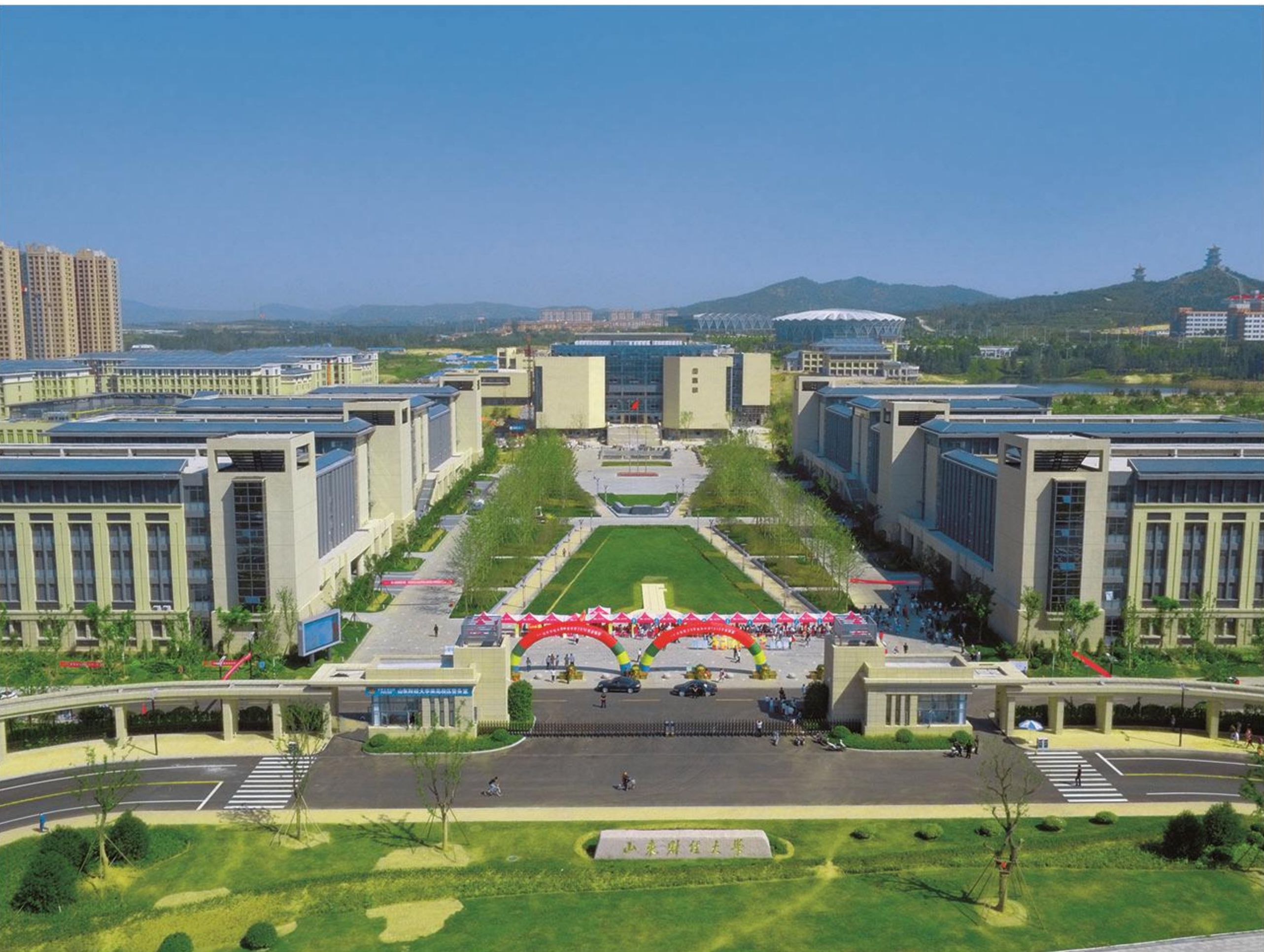
山东财经大学莱芜校区项目（国内高校首个资产证券化项目） Shandong University of Finance and Economics - Laiwu Campus (first asset securitization project in China's universities)
