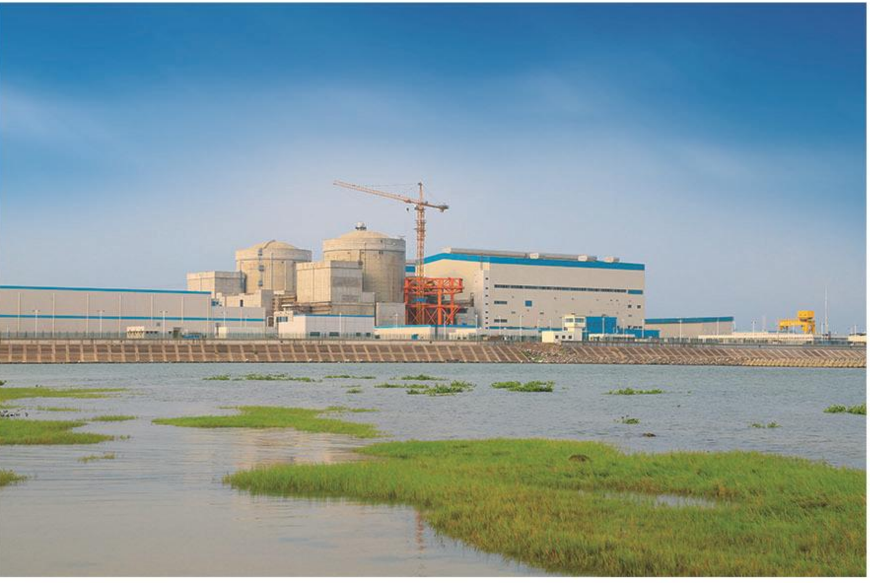
辽宁红沿河核电站，东北第一座核电站 Liaoning Hongyanhe Nuclear Power Plant, the first nuclear power plant in Northeast China
