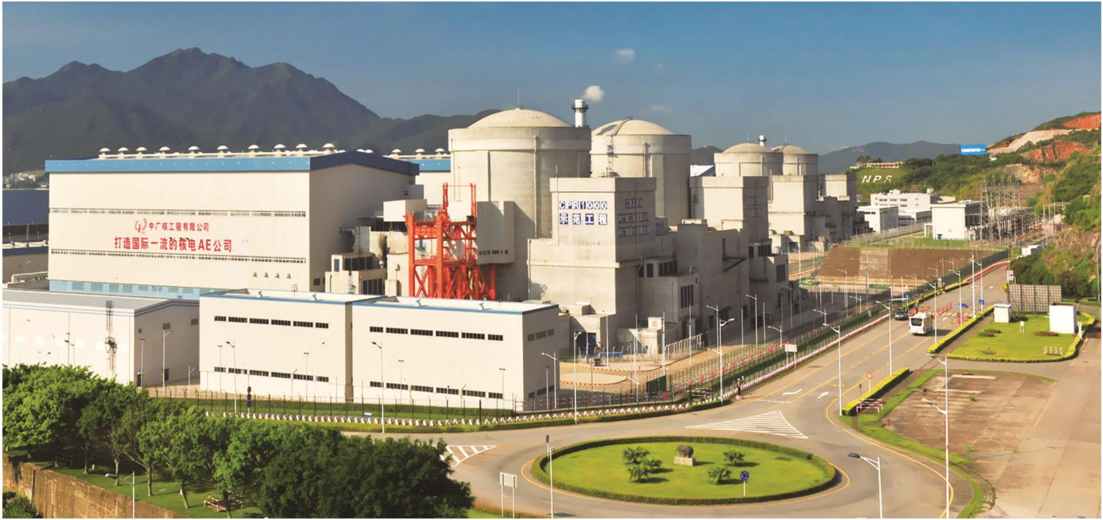
广东岭澳核电站 CPR1000堆型，建筑工程鲁班奖 Guangdong Ling'ao Nuclear Power Plant CPR1000 Reactor, Construction Engineering Luban Award
