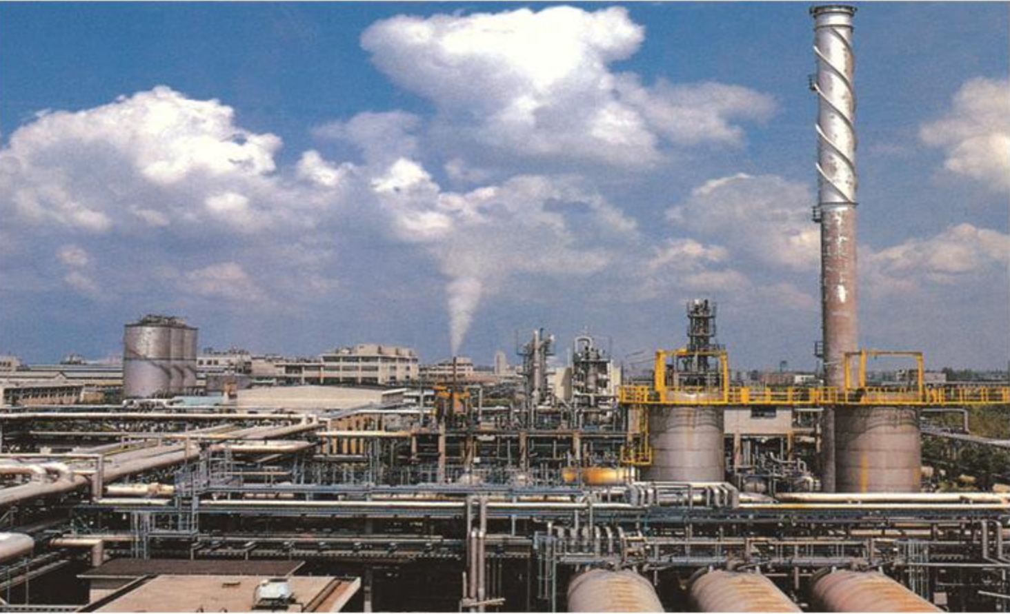
仪化50万吨/年大容量聚酯项目（设计+监理） Yihua 500,000 tons / year Large Capacity Polyester Project (Design + Supervision)
