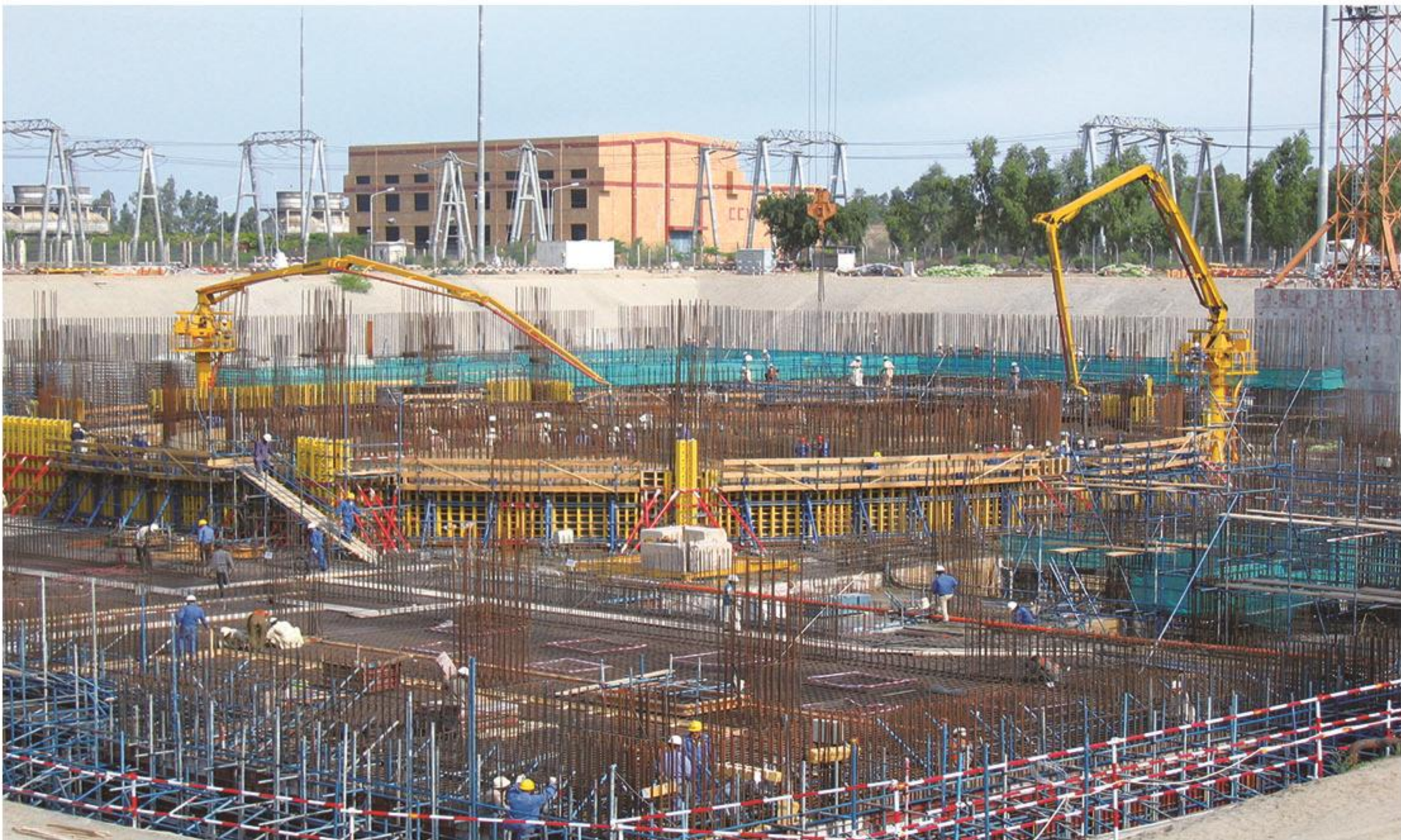
核岛筏基整体浇注 Pouring of entire nuclear island raft foundation
