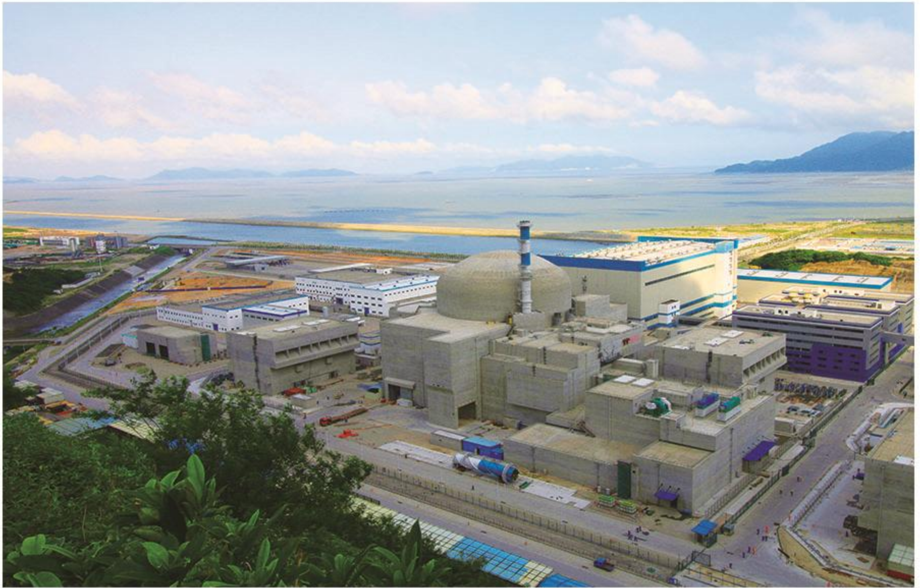
广东台山核电站 EPR全球首堆，全球单机容量最大 Guangdong Taishan Nuclear Power Plant EPR - the world's first reactor, with the world's largest single unit capacity
