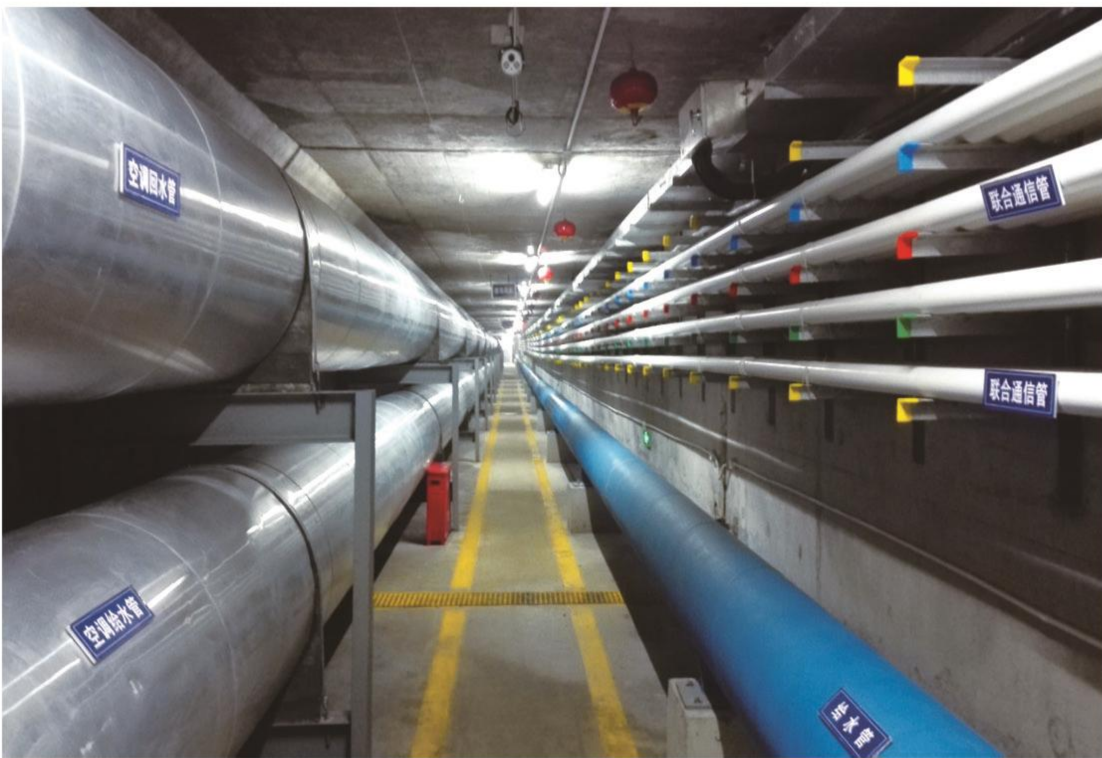
地下综合管廊施工 Underground integrated pipe gallery construction
