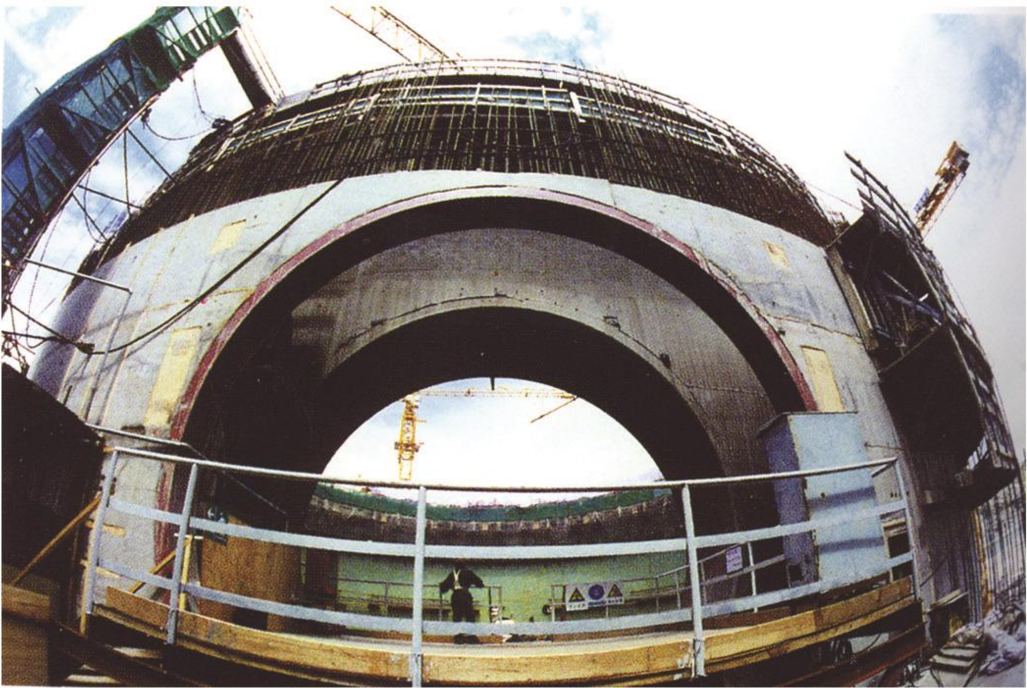
核岛双安全壳施工 Nuclear island double containments construction
