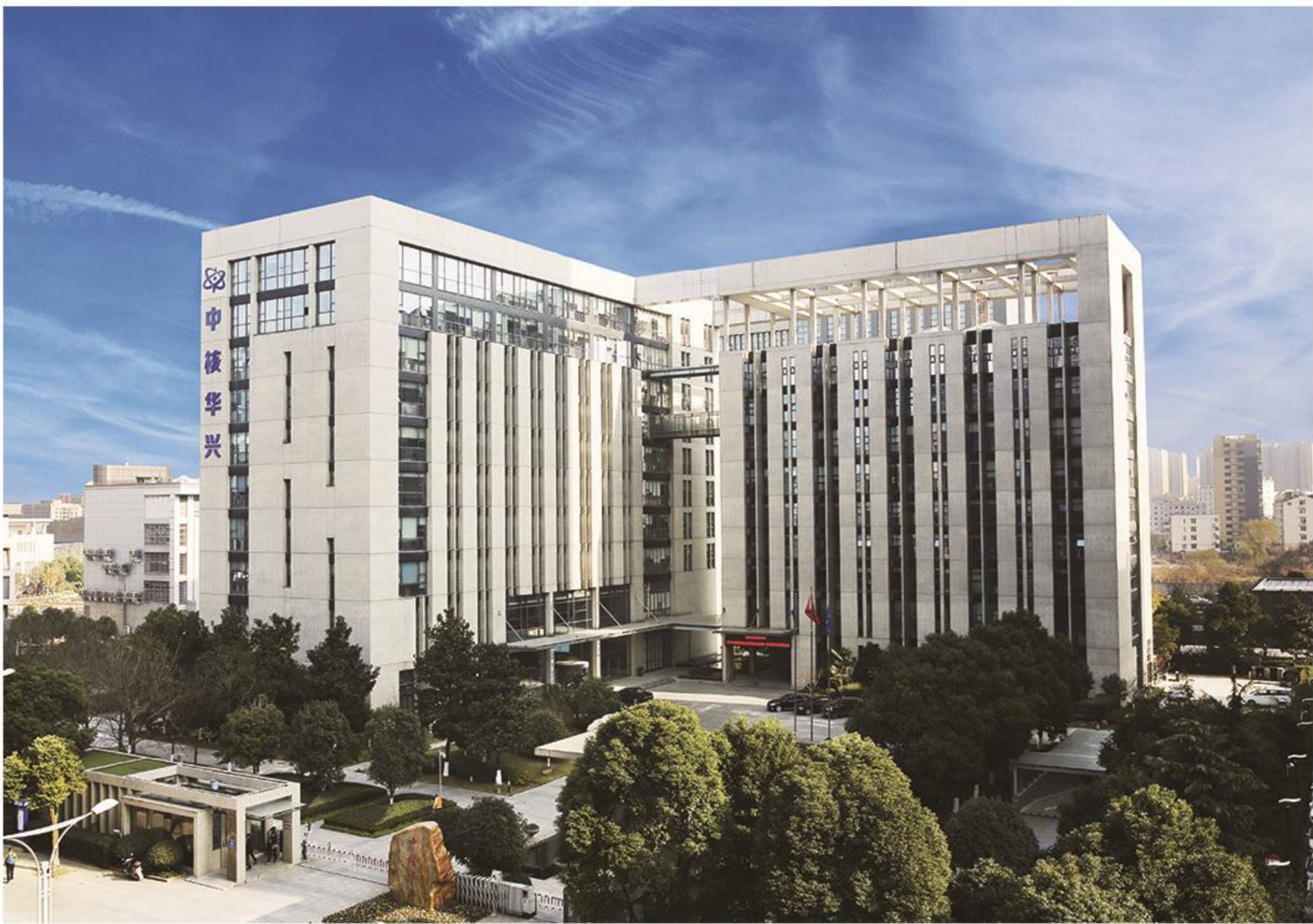
清水混凝土施工 Fair-faced concrete construction
