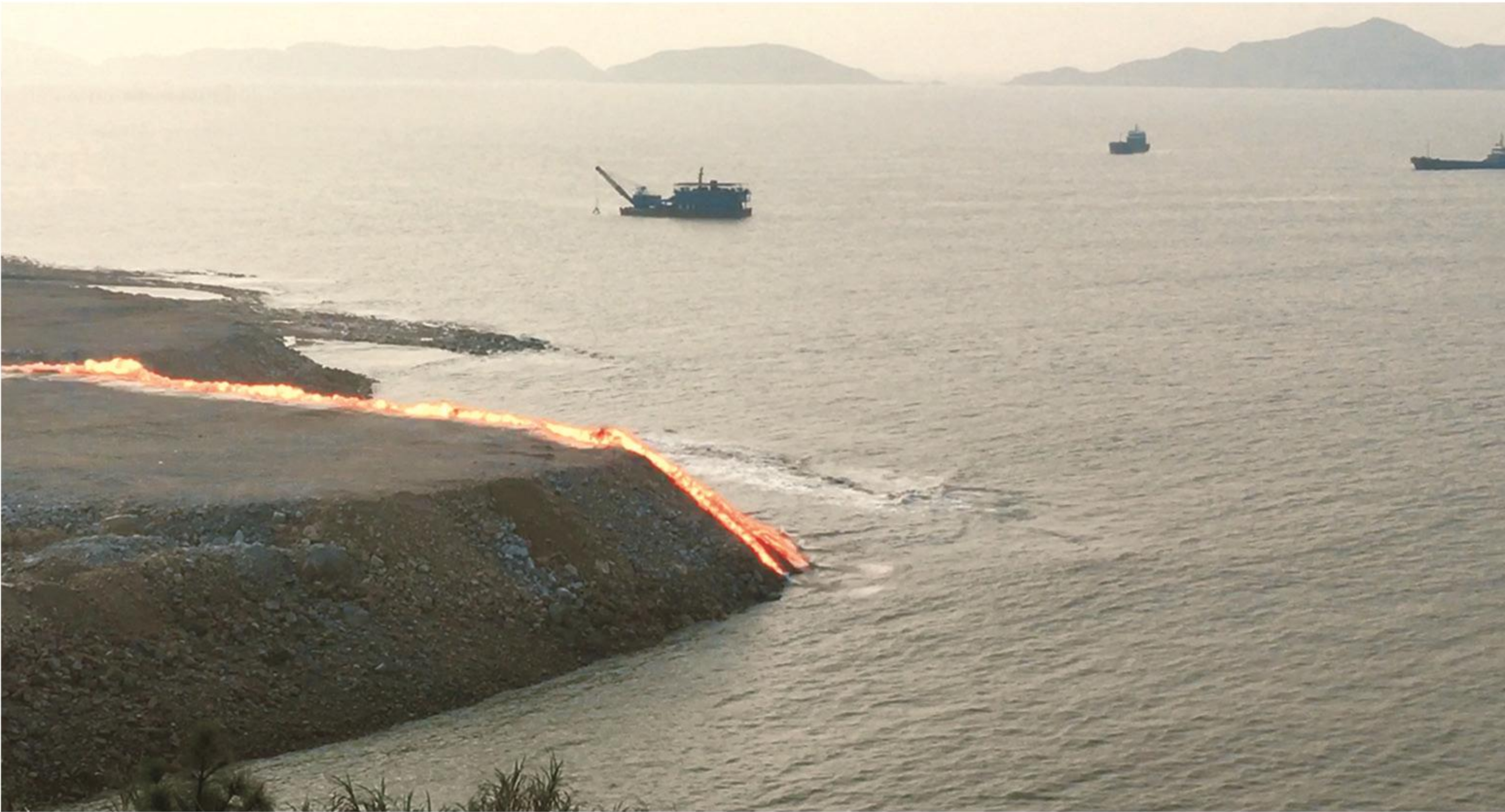
超深厚淤泥爆破挤淤 Ultra-deep sludge blasting and squeezing
