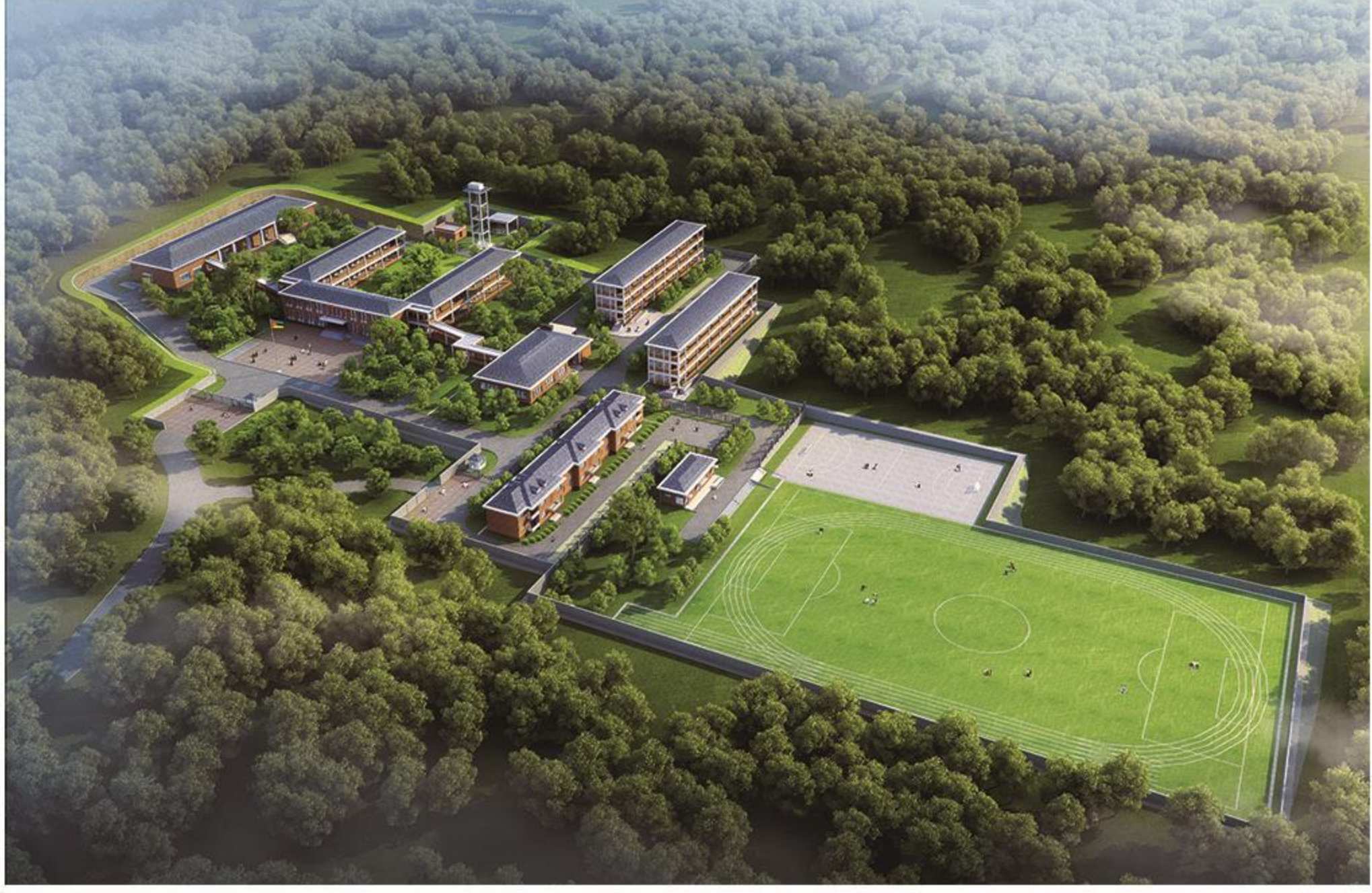
援莫桑比克索法拉职业技术学校项目 Assistance Mozambique Sofala Vocational and Technical School Project
