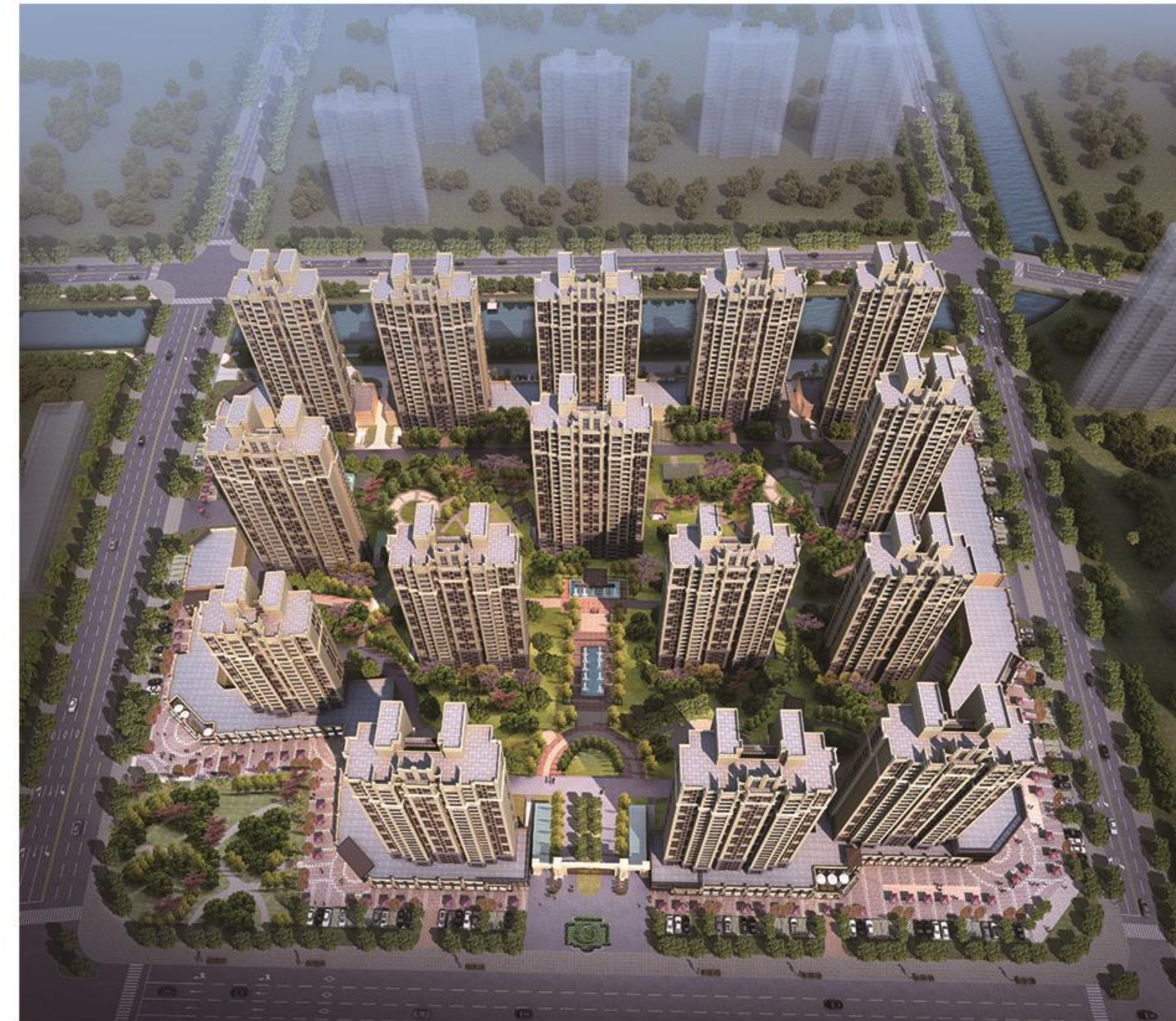
鄞县政府片区安置房EPC项目 EPC Project of Resettlement House in Juancheng County Government Area
