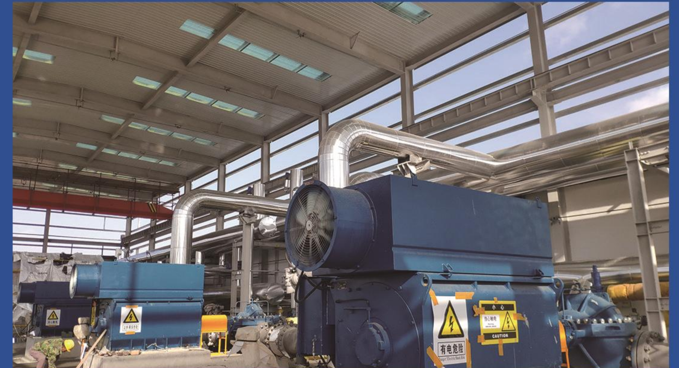
甘肃省金昌市永昌县热电联供项目 Combined heat and power project in Yongchang County, Jinchang City, Gansu Province
