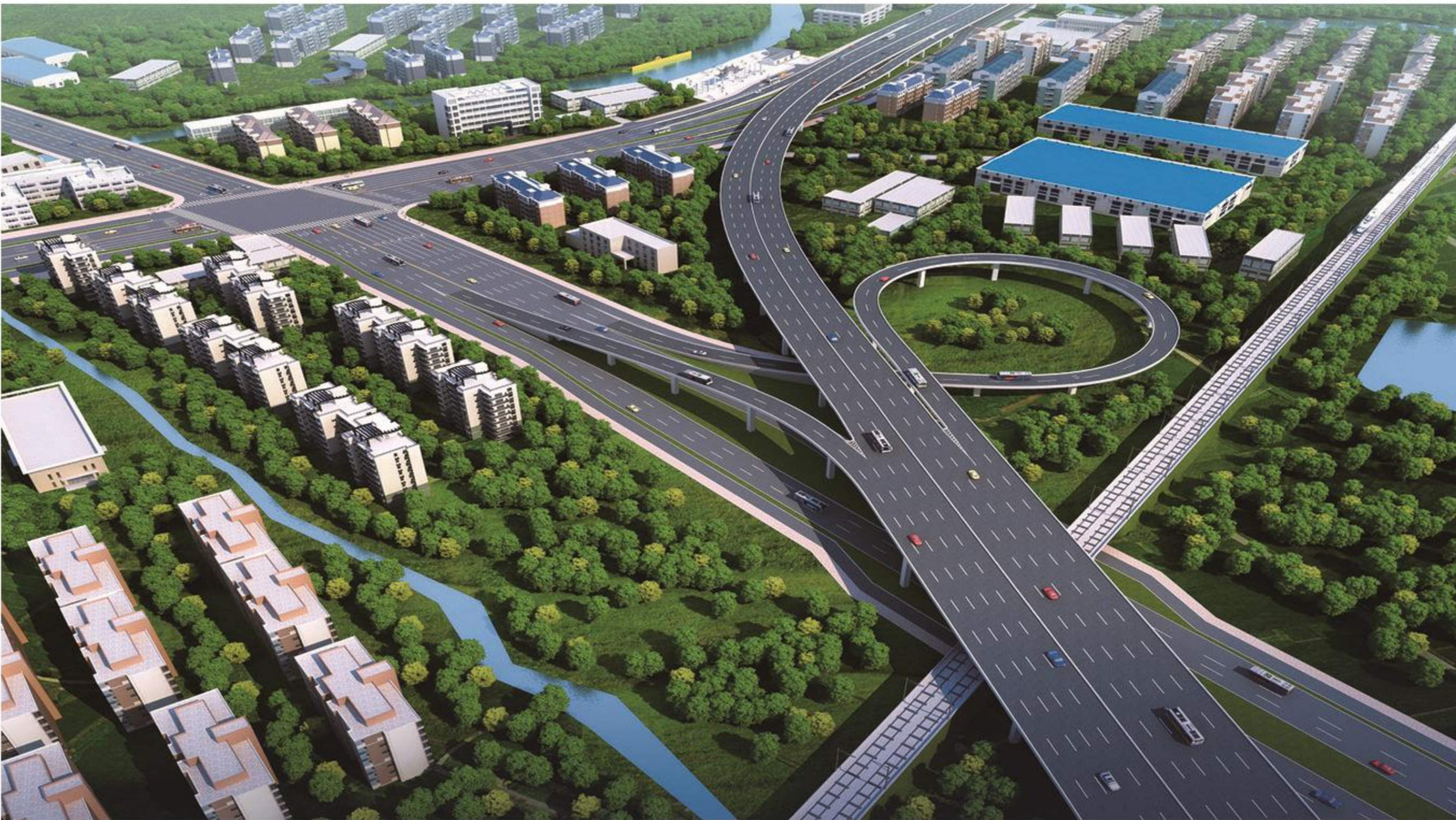
大型公路、市政工程施工 Large-scale highway and municipal engineering construction
