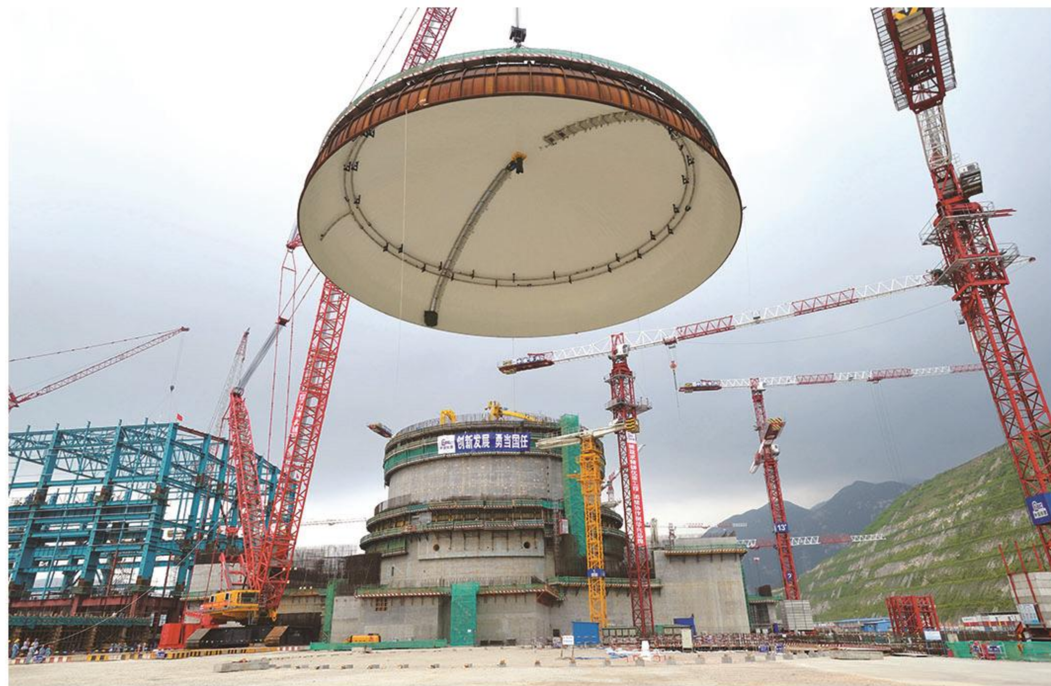
穹顶整体吊装技术 Overall lifting technology of the dome
