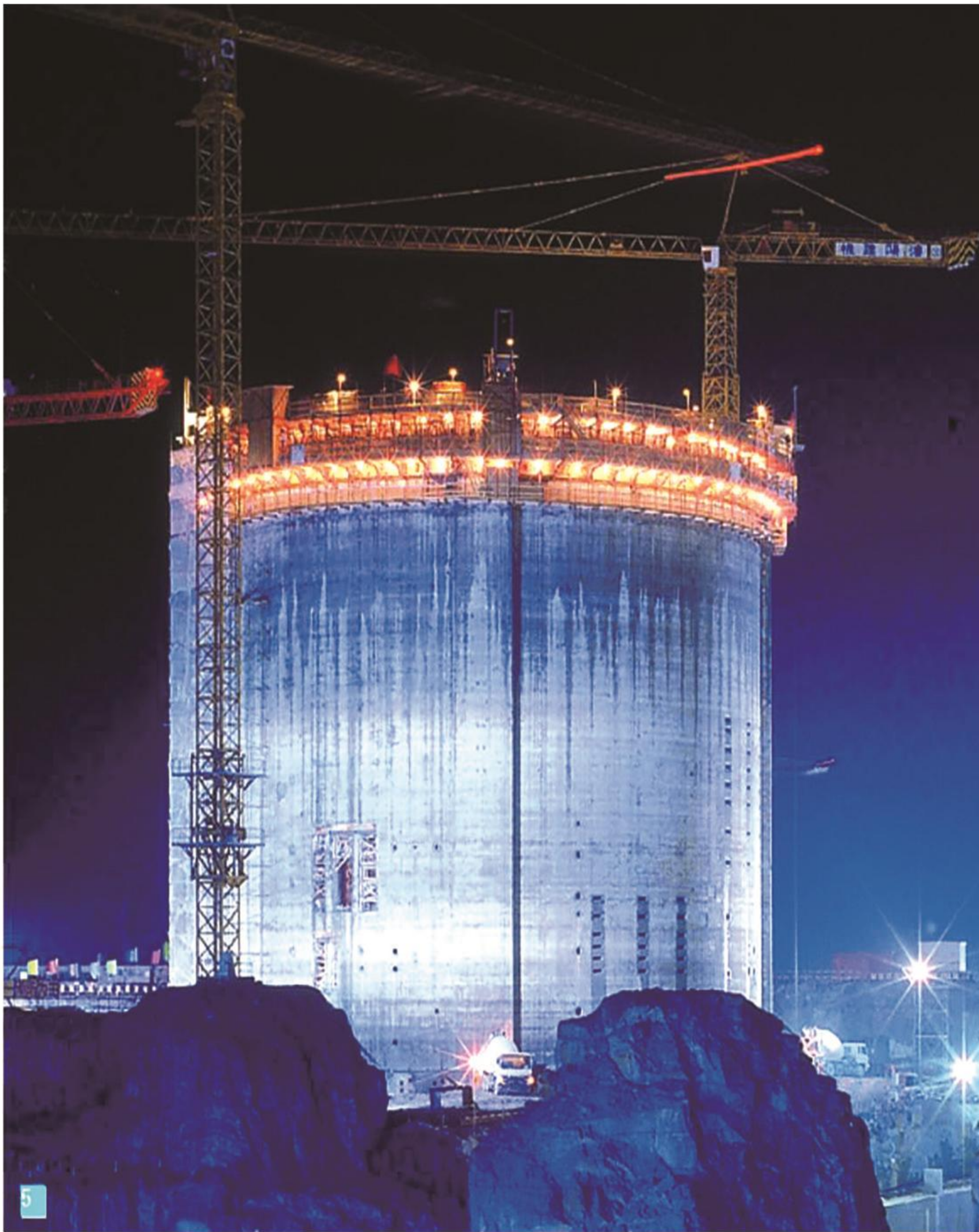
核岛滑模施工 Nuclear island slip-form construction
