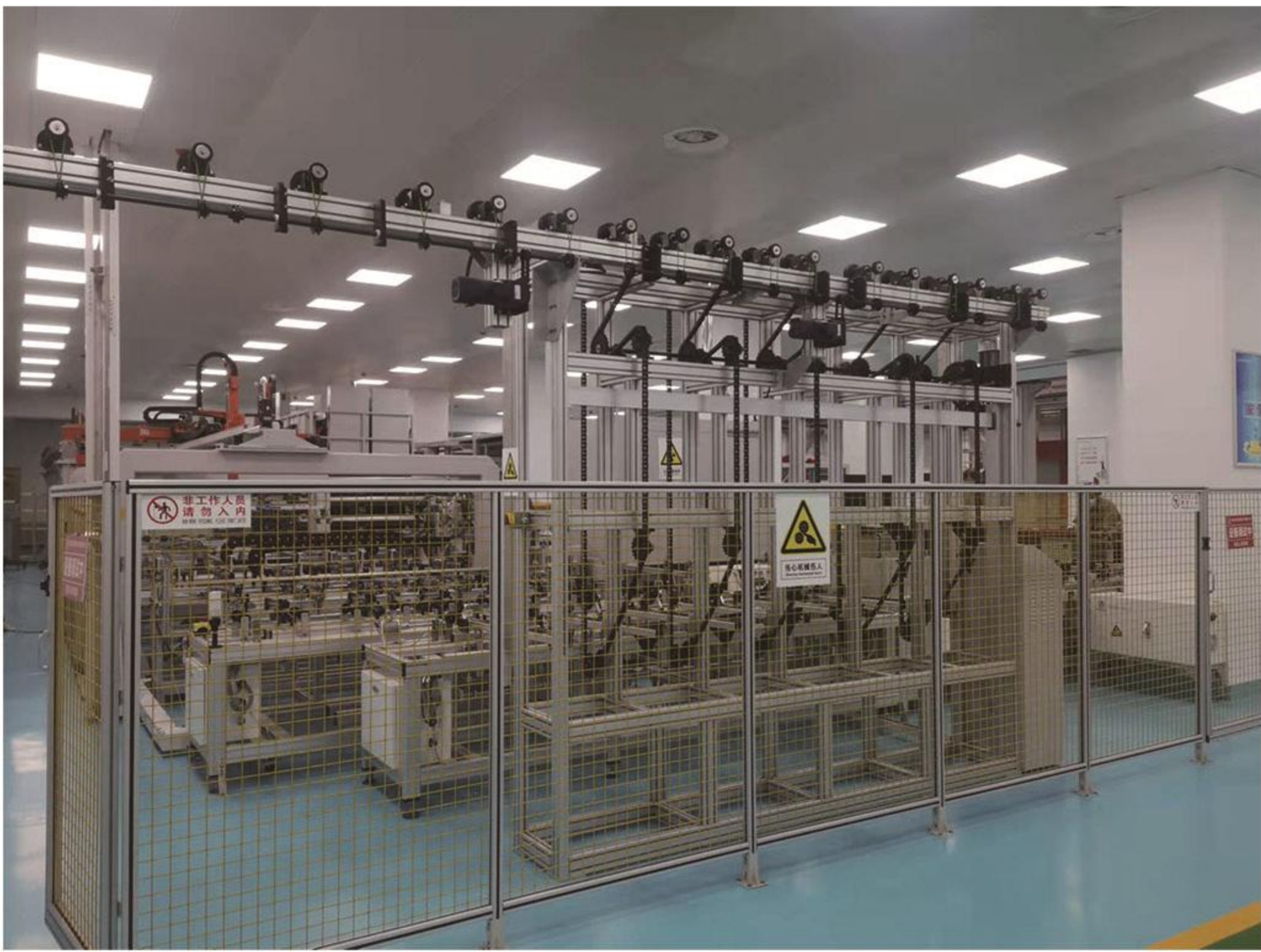
核燃料生产线设备安装施工 Equipment installation and construction of nuclear fuel production line
