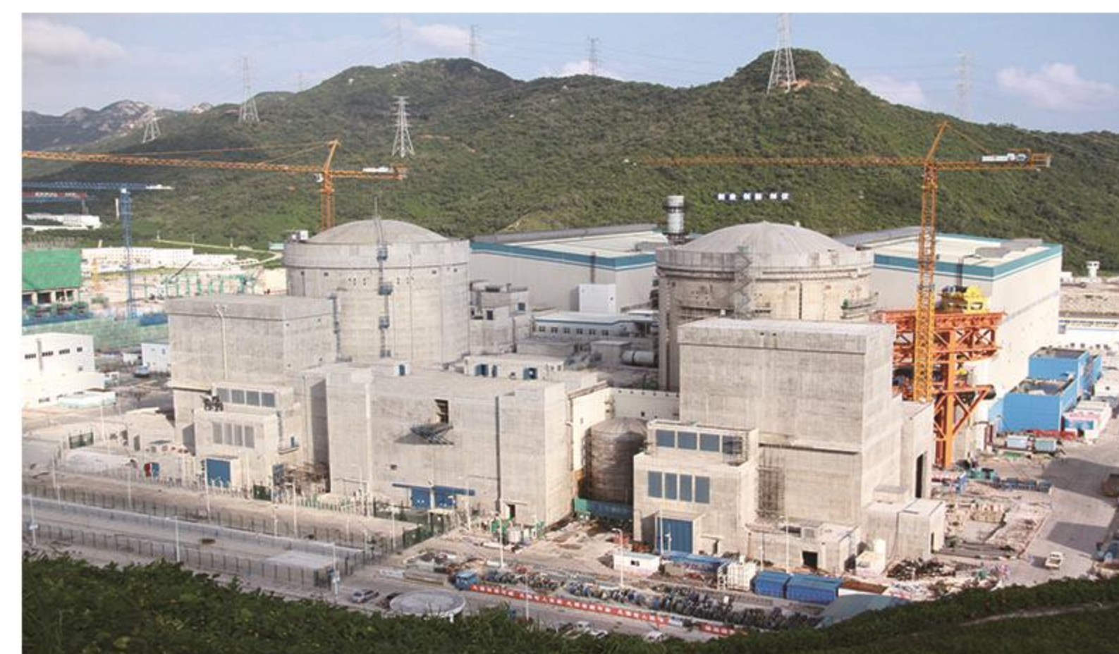
阳江核电3、4号机组（国家优质工程金奖） Units 3 and 4 of Yangjiang Nuclear Power Plant (Golden Medal of National High Quality Project)
