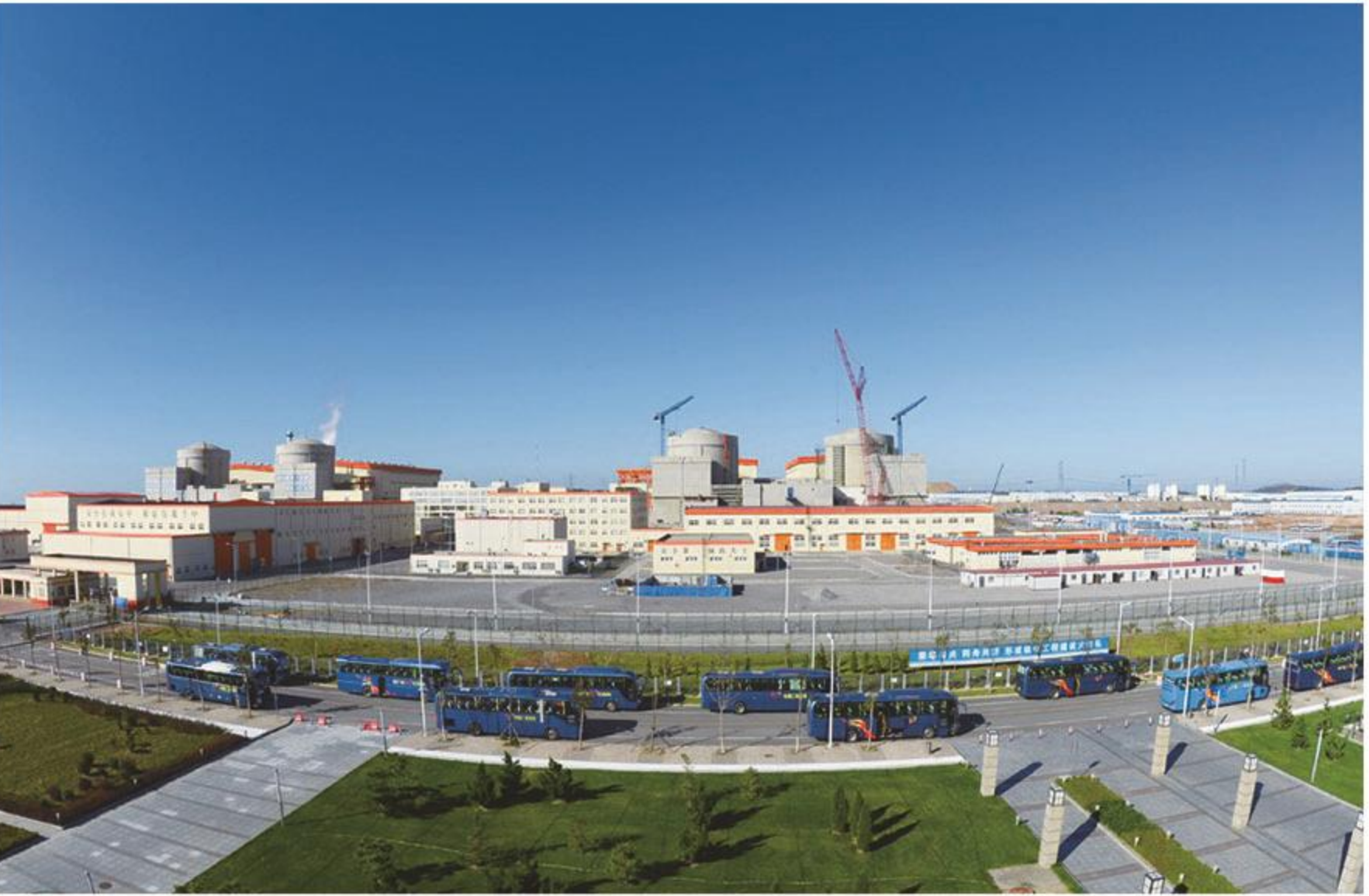
广西防城港核电站，西部第一座核电站 Guangxi Fangcheng Port Nuclear Power Plant, the first nuclear power plant in West China
