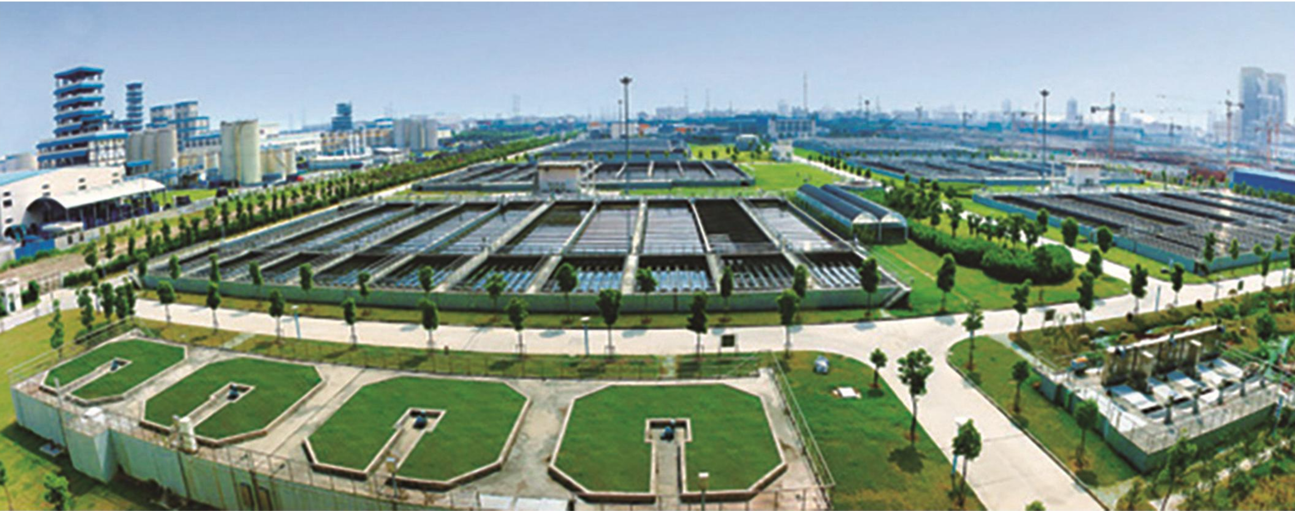
上海白龙港污水处理厂项目 Shanghai Bailonggang Sewage Treatment Plant Project
